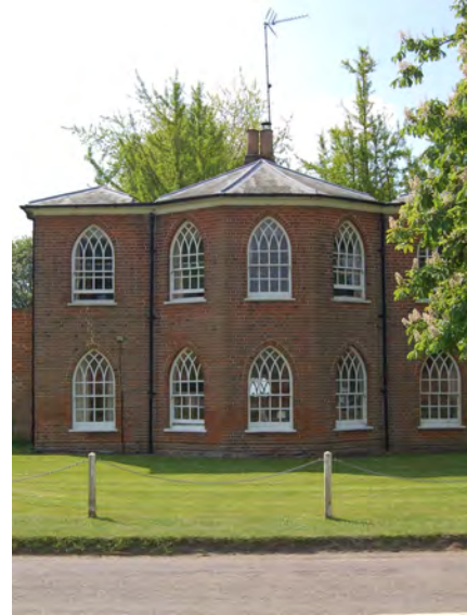
Picture 1.4 Elegant 'Gothick' 2-centred arched form windows are employed to dramatic effect on Lion House.
