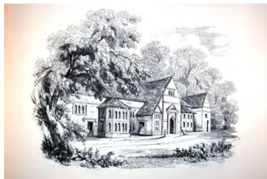
Picture 1.25 A view of the back of the stable block as it appeared in 1836, from Richard Neville's 'History of Audley End'.
