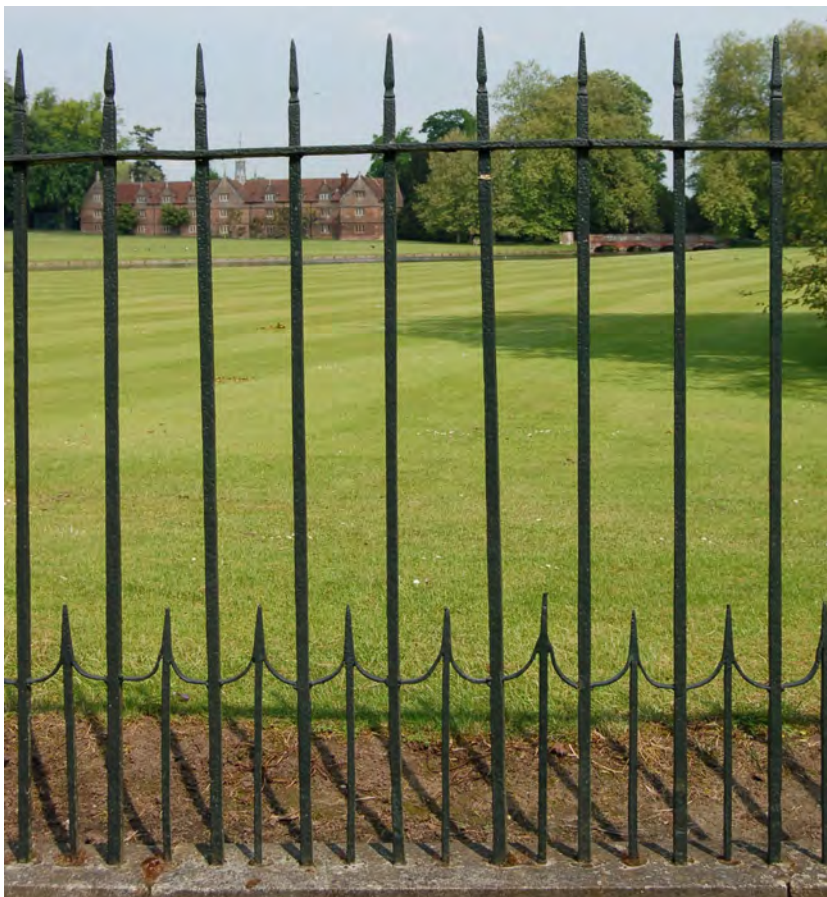
Picture 1.6 Fine early 19th century square section iron railings define the south boundary of Audley End Park.
