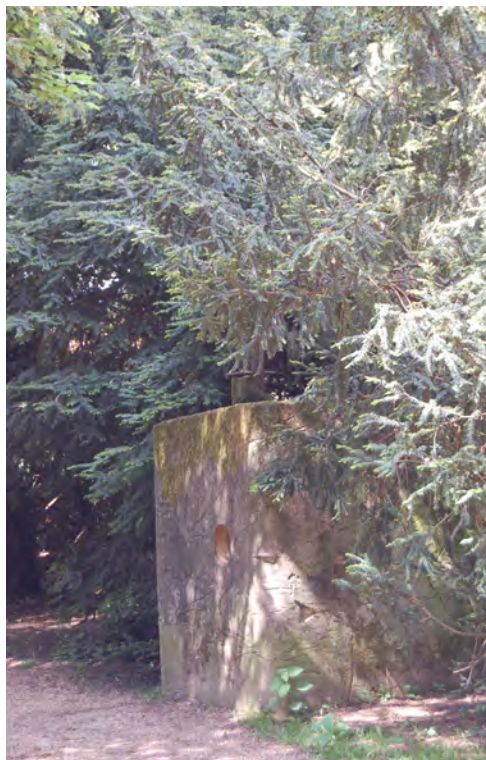
Picture 1.30 Road block located immediately to the west of the Fly Bridge.
