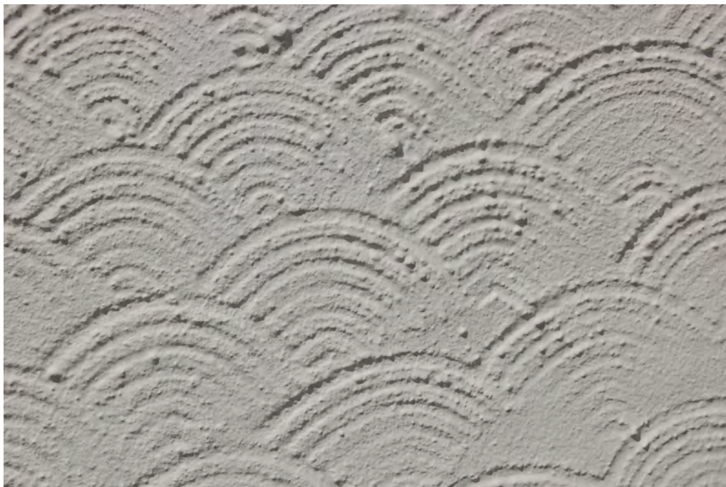
Picture 1.2 Traditional Essex combed pargetting within panels on the wall of one of the estate cottages in Audley End Village.
