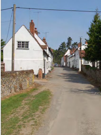
Picture 1.18 Overhead services on utility poles are somewhat disruptive in the streetscene.
