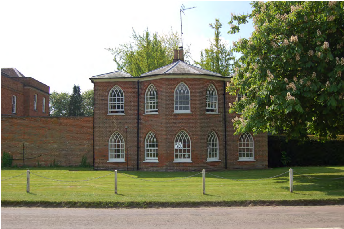
Picture 1.15 The visually arresting prospect of Lion House with its range of 'Gothick' windows, set back from the road and framed by mature horse chestnuts.
